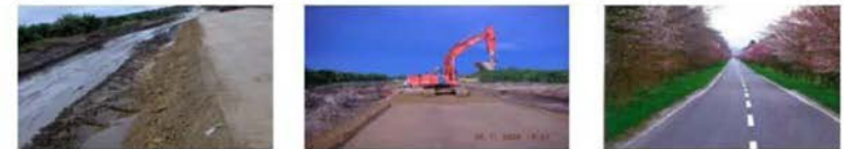
Malaysia subbase and the surface layer (Bintulu)
