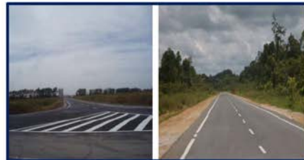
(COMPLETED UP TO SUB-BASE BY T-GSC)
